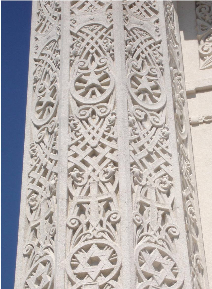
Closeup of ornamentation on exterior pillar
